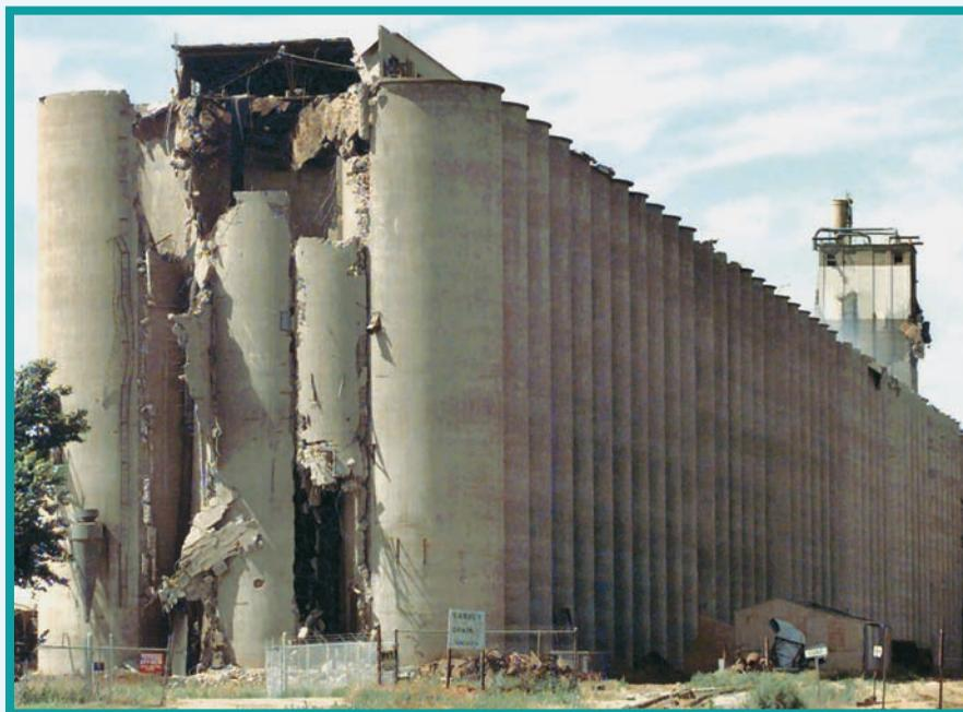
**Figure 5.1** A grain explosion caused the damage to this grain mill.
